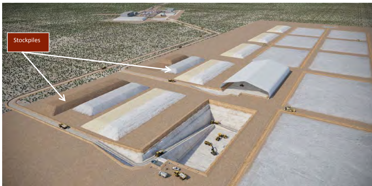
Figure 5-7 Stockpiles adjacent to pits/cells
