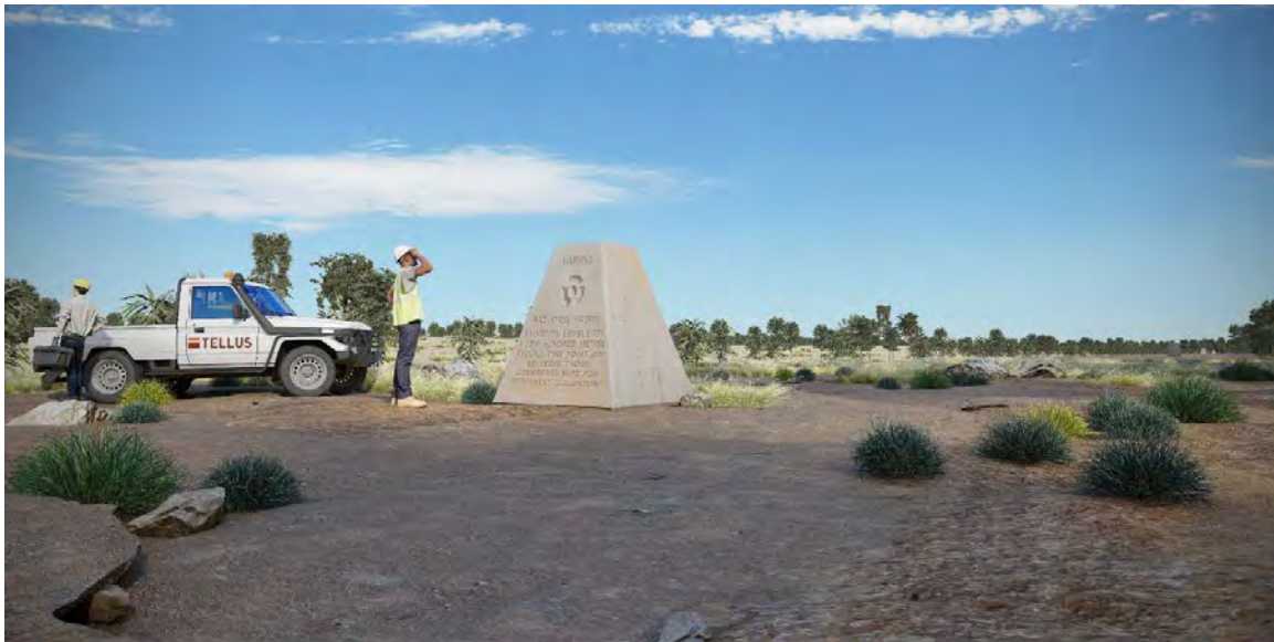
Figure 10-7 Example of surface monument indicating a change in land use
