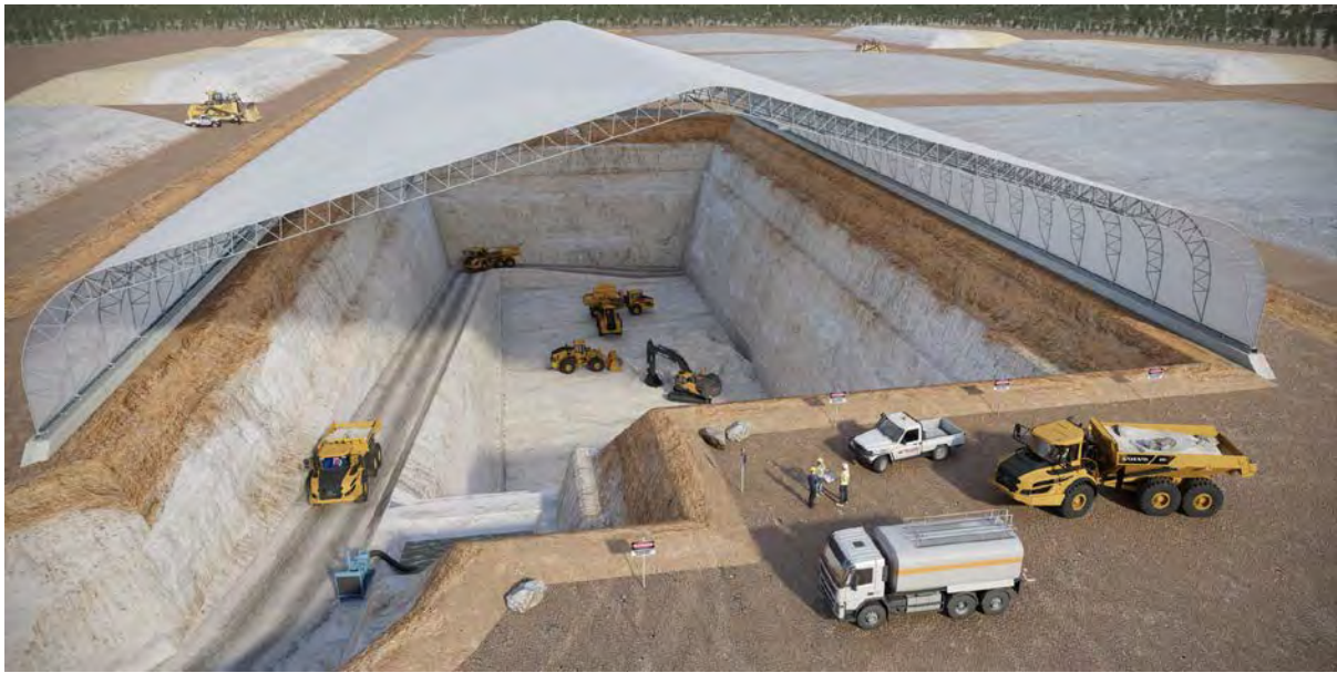
Figure 5-5 Conceptual view of pit being mined and pit with roof canopy
