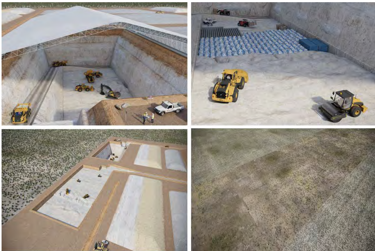
Plate 1-2 Process of creating the kaolin open cut pit, filling it with waste materials, and then undertaking remediation and closure
